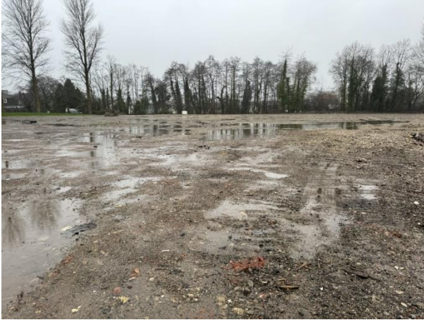
Photo 7: Bare ground within the centre of the development site
