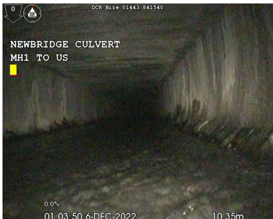
Figure 2-3 CCTV survey of box culvert below Site
