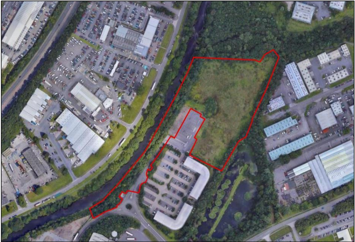
Figure 3. Aerial image of site showing habitats: Bare Ground, Marshy Grassland, Treeline, Scrub within the wider habitats of Wooded belts, Native Broadleaved Woodland, watercourses, and waterbodies.
