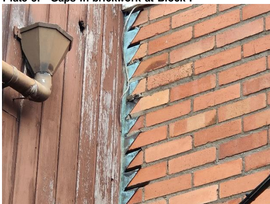
Plate 5: Gaps beneath boarding on southern elevation of block F
