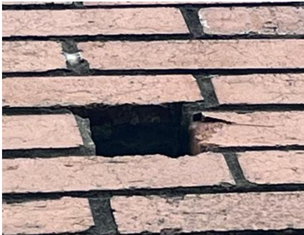
Photo 59: Missing Brick, Eastern Elevation (J Block)
