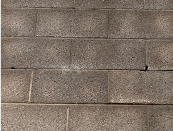
Photo 35: Cavities in Mortar (C Block)
