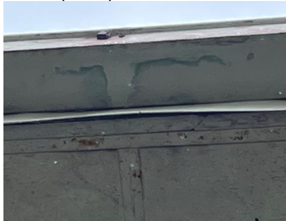
Photo 54: Gaps Beneath uPVC Trim, Southern Elevation (G Block)
