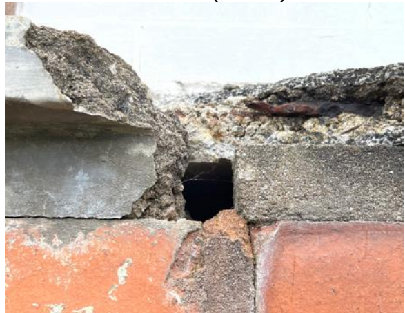
Photo 48: Eroded Mortar (G Block)
