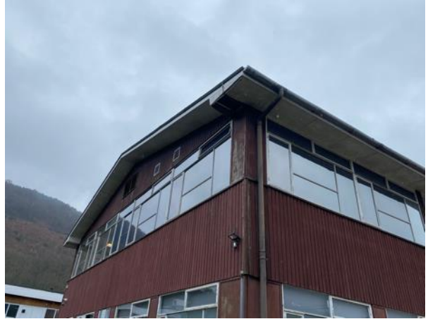
Photo 64: Large Missing Section of Soffit (K Block)
