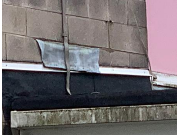
Photo 76: Gap Beneath Roofing Felt (T Block)
