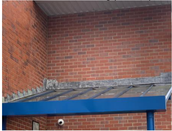
Photo 72: Gap in Trim of Soffit (Block L/R)
