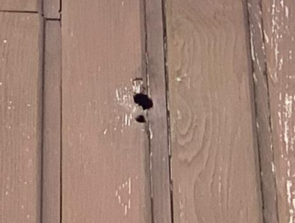
Photo 29: Large Gap in Soffit Box (B Block)
