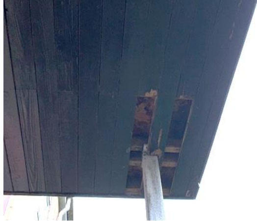
Photo 82: Vents Present (Guarding Unknown) (T Block)
