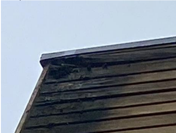
Photo 89: Gap in Wall Above Flat Roof (X Block)
