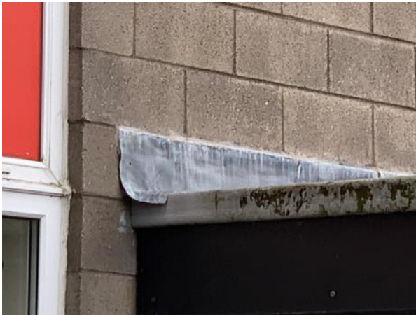
Photo 77: Lifted Lead Flashing (T Block)
