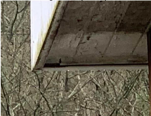
Photo 95: Damaged Timber Soffit (Z Block)
