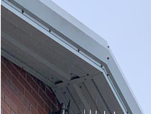
Photo 71: Gaps Present in Soffits at Apex (Block L/R)
