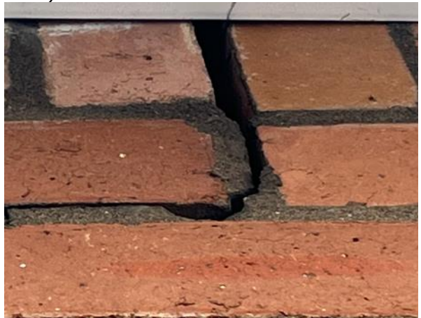
Photo 40: Gaps in Brickwork Beneath Soffit (E Block)
