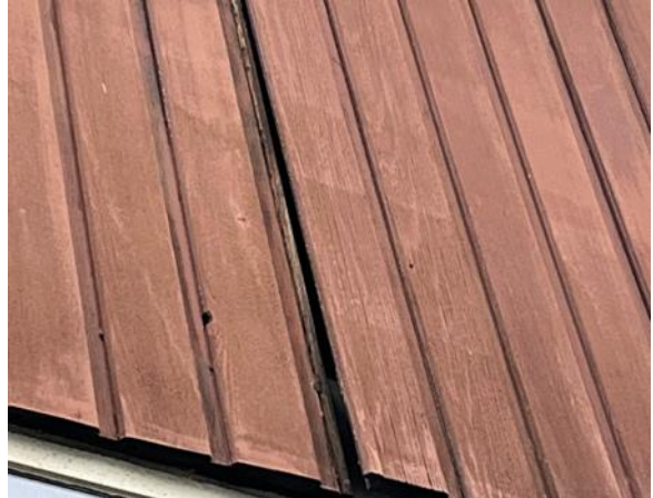
Photo 46: Damaged Wood Panelling (F Block)
