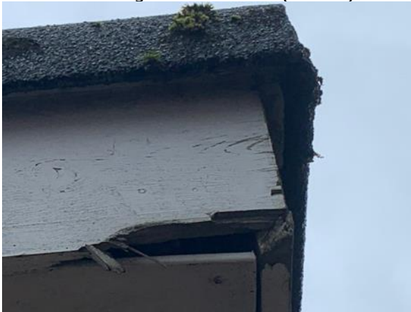
Photo 95: Damaged Timber Soffit (Z Block)
