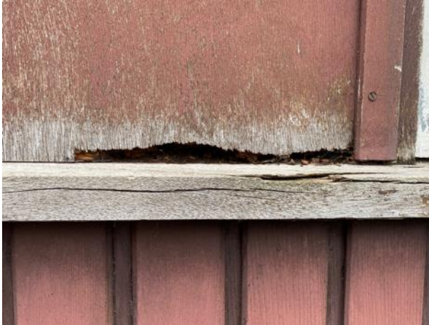
Photo 65: Damaged Wooden Panelling (K Block)
