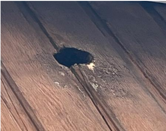
Photo 41: Crack in Plastic Soffit Trim (E Block)
