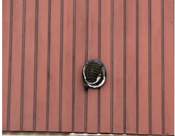
Photo 66: Uncapped Vent (K Block)
