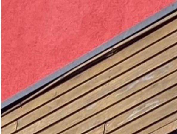
Photo 87: Damaged/Rotting Timber Panelling (X Block)
