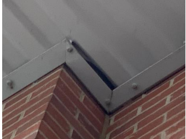
Photo 72: Gap in Trim of Soffit (Block L/R)
