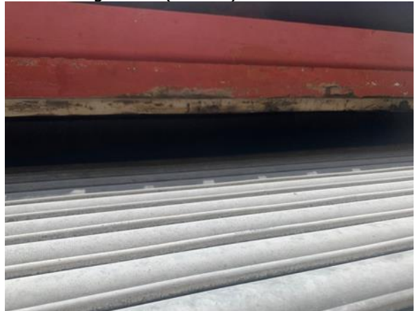
Photo 22: Gap Between Window Frame and Soffit Box (A Block)
