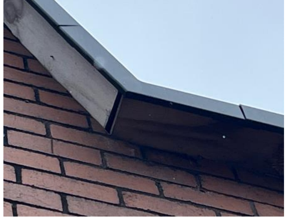
Photo 58: Gaps in Ridge/End Tiles (J Block)
