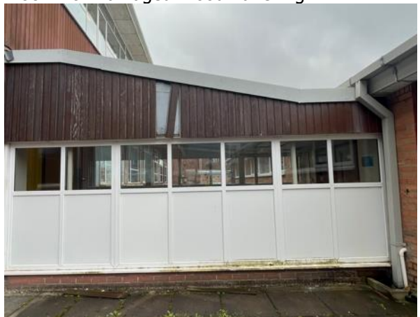
Photo 42: Connecting Building Between E and F Block with Damaged Wood Panelling
