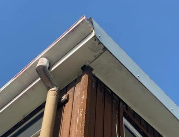
Photo 30: Gap in Soffit Box (B Block)
