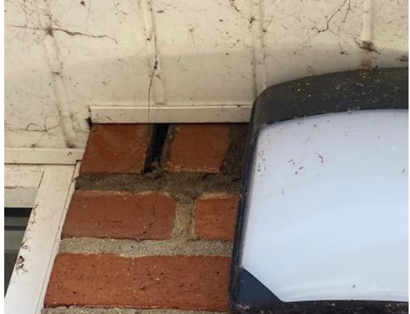
Photo 34: Small Cavity in Mortar (C Block)
