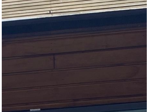
Photo 88: Lifted Wooden Panelling (X Block)
