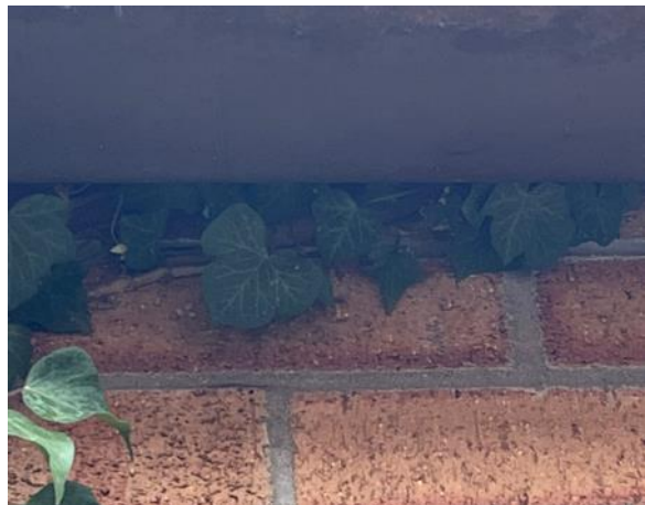
Photo 54: Gaps Beneath uPVC Trim, Southern Elevation (G Block)
