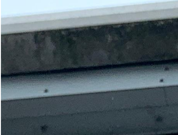
Photo 81: Raised Lead Flashing (T Block)
