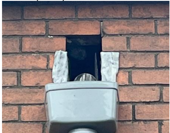
Photo 60: Gap Above Drain Pipe, Northern Elevation (J Block)
