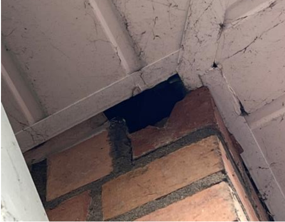
Photo 39: Hole in Wood Panelling (E Block)
