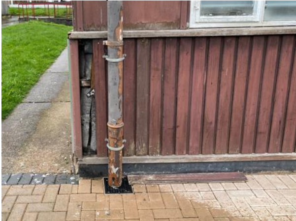
Photo 65: Damaged Wooden Panelling (K Block)
