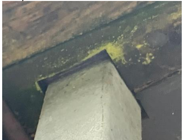
Photo 78: Gap in Porch Surrounding Pillar (T Block)
