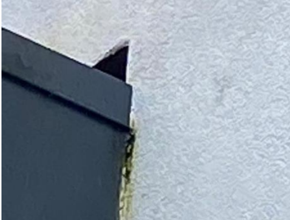
Photo 89: Gap in Wall Above Flat Roof (X Block)
