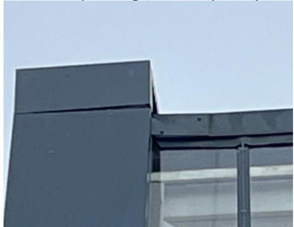
Photo 58: Gaps in Ridge/End Tiles (J Block)
