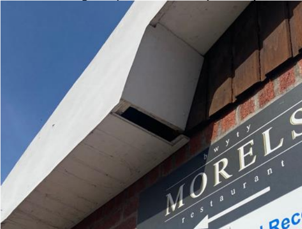
Photo 29: Large Gap in Soffit Box (B Block)
