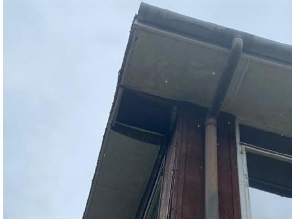
Photo 66: Uncapped Vent (K Block)
