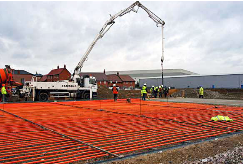
Installation of thermal bank under slab
