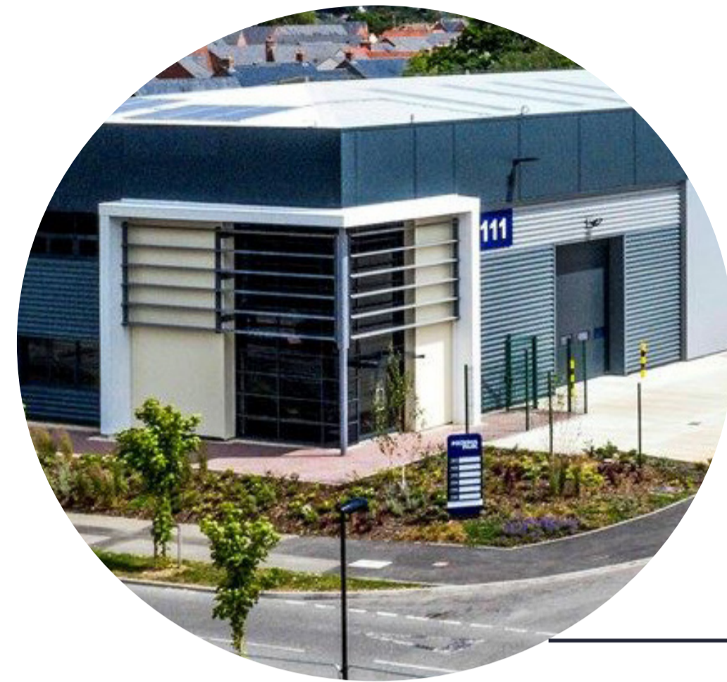
Building Frontage Create an attractive and functional development with identity, which relates well within its context.
