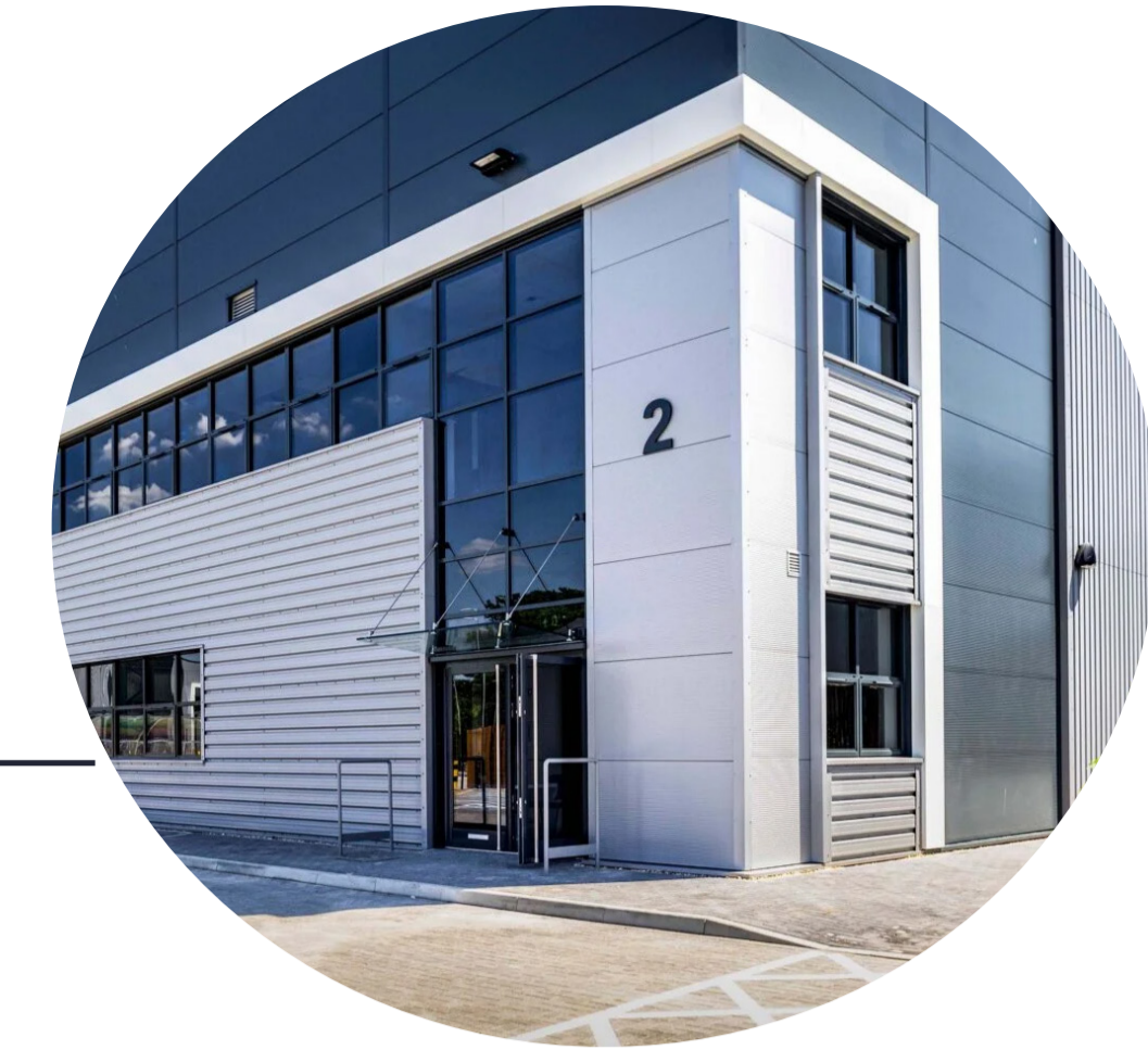
Office Frontage Well-designed, with attention to detail and provide clear legibility in the choice of façade material specifications.
